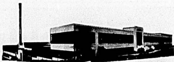
MAIN OFFICE AND PLANT: North Bergen, New Jersey
